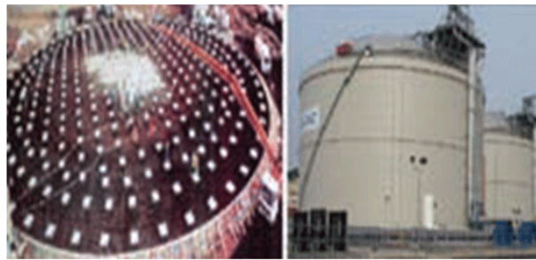
Figure 7: Proper layout of the reservoirs, considering the radius of the work with the radial structure of the basic separators [8]
