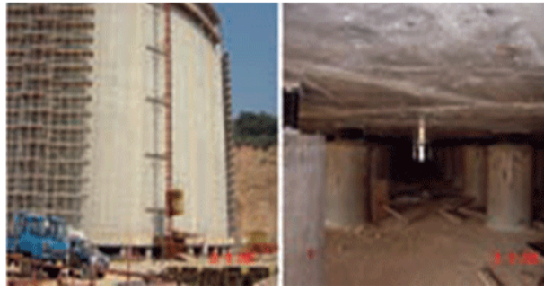
Figure 6: Basement Stabilization of Reservoirs by Using Basic Separators against Dynamic Load [6]
