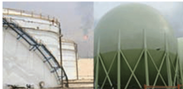
Figure 4: Misplaced layout of reservoirs and the possibility of the vulnerability of all reservoirs to the initial damage in one of them or due to the proximity of the explosion to the location of reservoirs [5]
