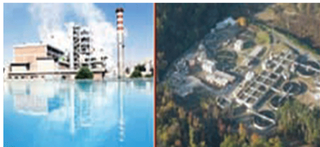
Figure 2: An example of a proper location in a vegetation shelter and incorrectly exposed [19]
