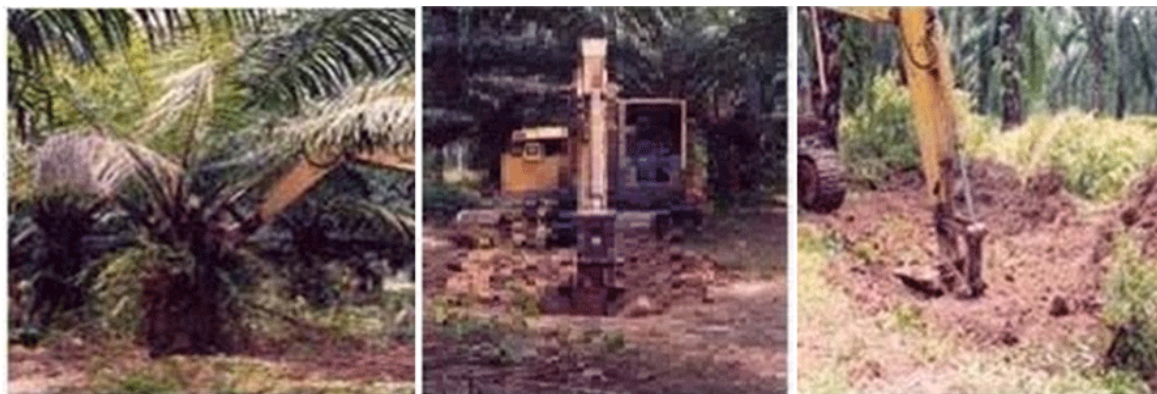
Plate 17: Control of BSR in existing stand by removal of diseased palm using excavator: pushing, excavating and refilling with nearby soil
