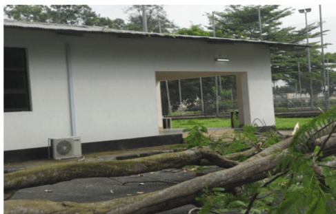
Plate 3: Tree fall by a residential building
